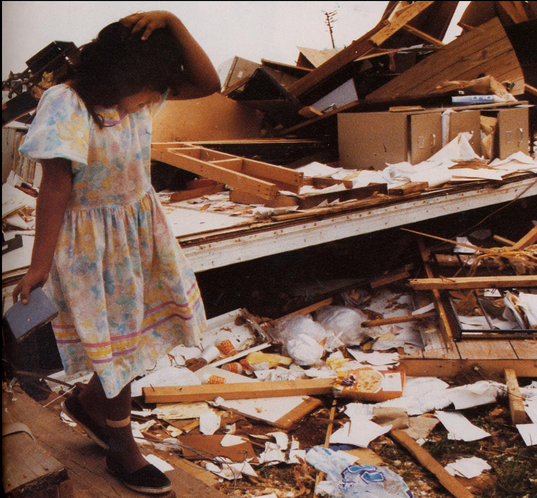
Child surveys home damage
